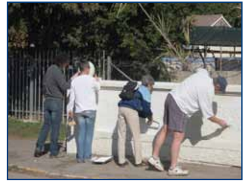
Staff members participate in the painting of the Kowie Ditch bridge
